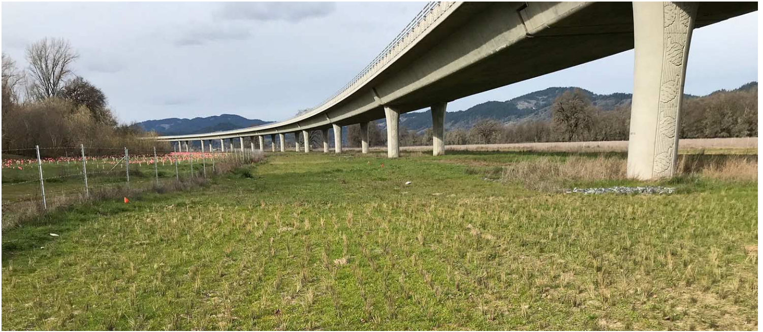
Riparian (pink flags in the background) and wetland restoration plantings (foreground) adjacent to the elevated viaduct of Willits Bypass.
