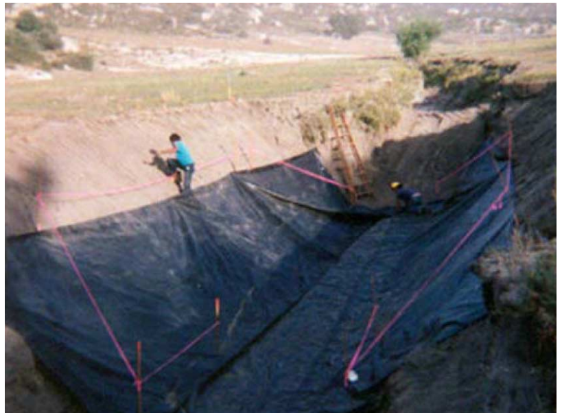
Geofabric liner in arroyo.
