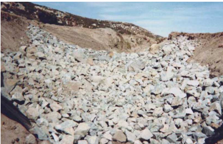
Piling of rip rap on fabric.
