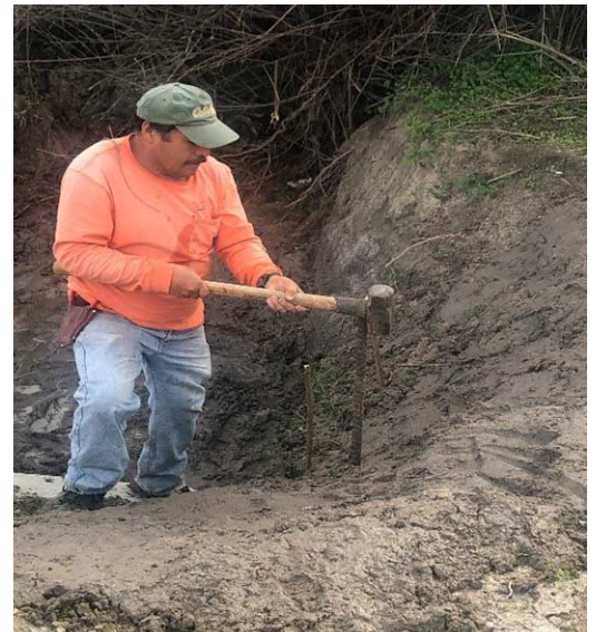
Habitat West Crew Member installing mulefat cuttings.
