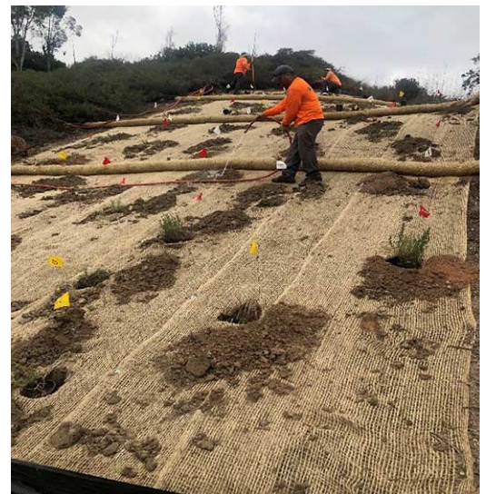
D&D Crew installing and watering plants
