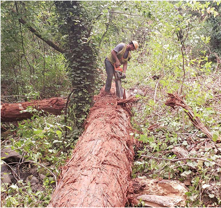
Log structures, installed below dam, used existing trees harvested onsite.
