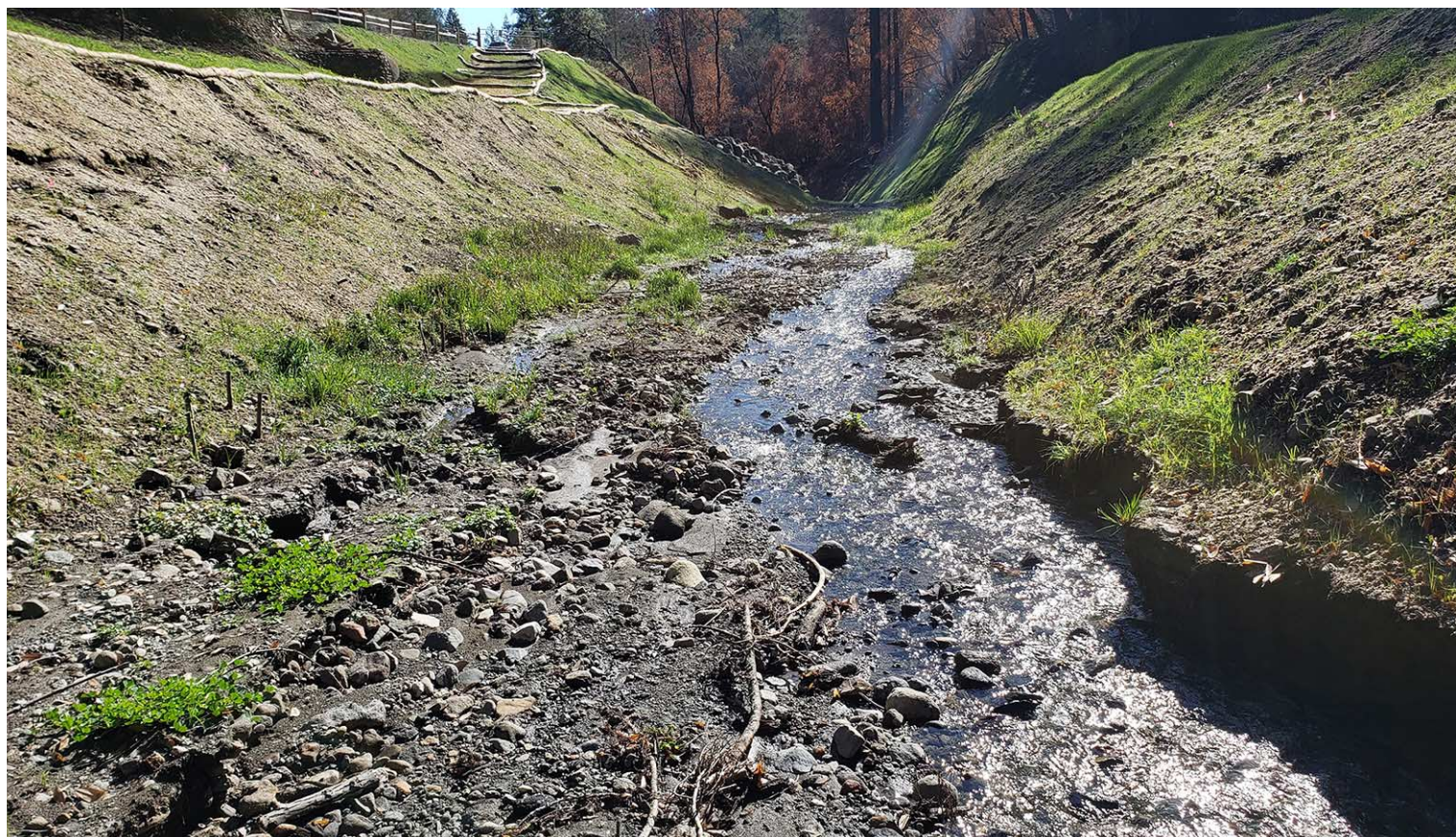
Low flow channel beginning to form in area of former reservoir.
