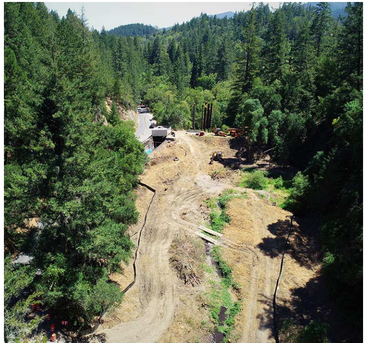
Upper York Creek Dam and reservoir cleared and ready for construction.
