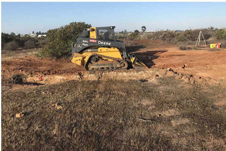
Vernal pool grading in action.
