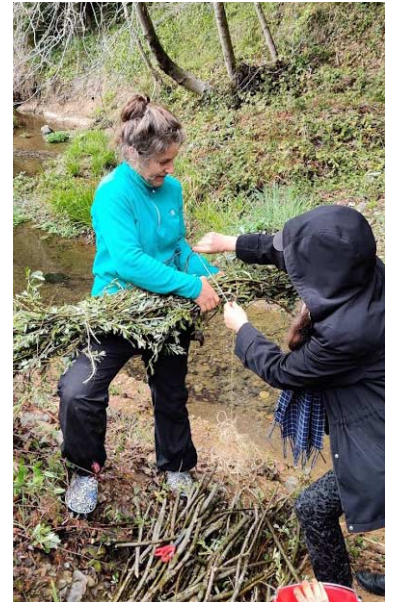
From left: On-contour, entrenched willow fascines (wattles) installed to naturally prevent erosion of a steepened creek bank and improve riparian habitat conditions. Illustration by Valerie Cepa. Live willow stake drawing from Groundwork: A Handbook for Small-Scale Erosion Control in Coastal California. Illustrated by Prunuske Chatham, Inc. and modified by Sarah Phillips. At a hands-on Marin RCD soil bioengineering workshop, landowner Katie Warfield learns how to secure a willow fascine for installation at the toe of her eroding creek bank in west Marin. Photo courtesy Sarah Phillips.
