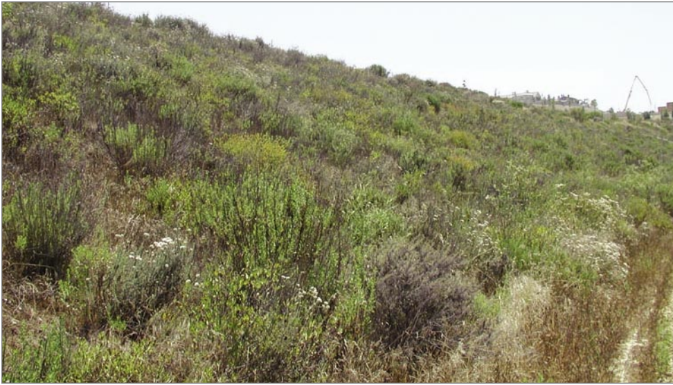
Five-year revegetated north slope of the Coyote Canyon landfill implemented with seeding only.
