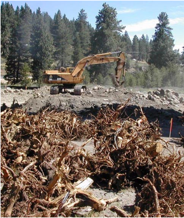
LEFT Stockpiled rootwads to be used in final grade.
